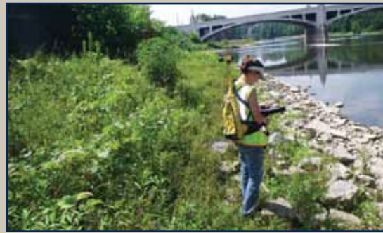
Two KCI crews spent 34 days in the field, inspecting 116 miles of levees, like the Wyoming Valley, Pa., system shown here, which included 2.5 miles of floodwall, 35 pump stations and approximately 1,000 drainage structures.
