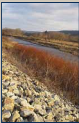
Prior to and during the inspections, KCI met the local sponsors including the Borough of Elkland, responsible for O&M for this 2.9-mile long flood risk management system in Pennsylvania.
